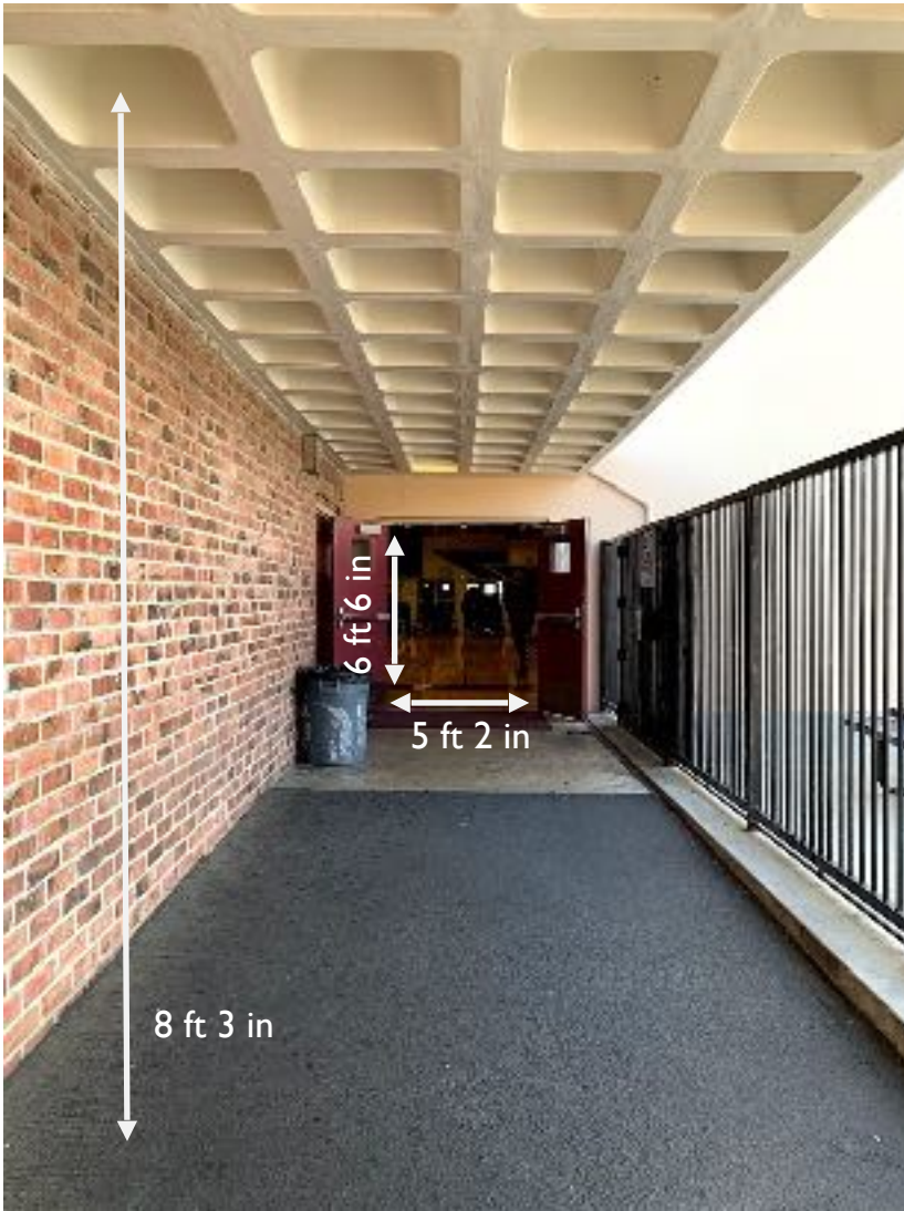
Corridor toward Ensemble Entrance
